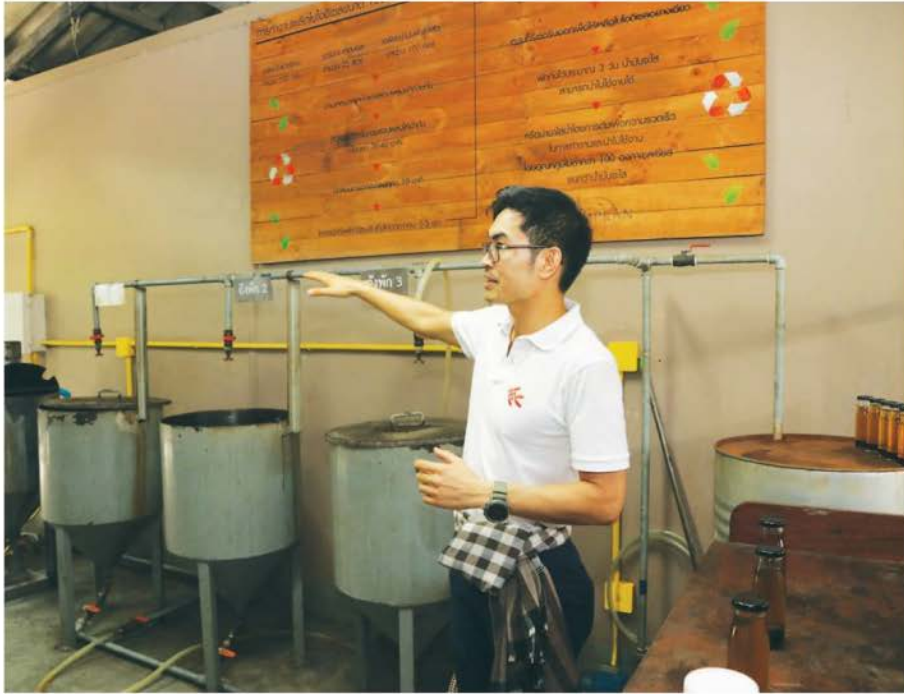
The bio-diesel plant at Sampran Riverside Hotel.
